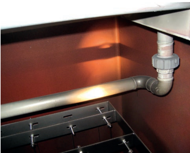
COROFLAKE coating in a wet ESP
