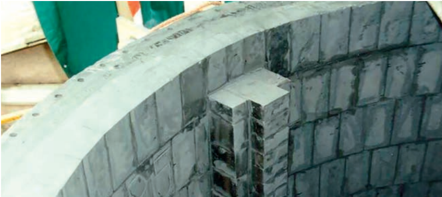
Vessel lined with carbon bricks and CHEMOKITT FU 1320
