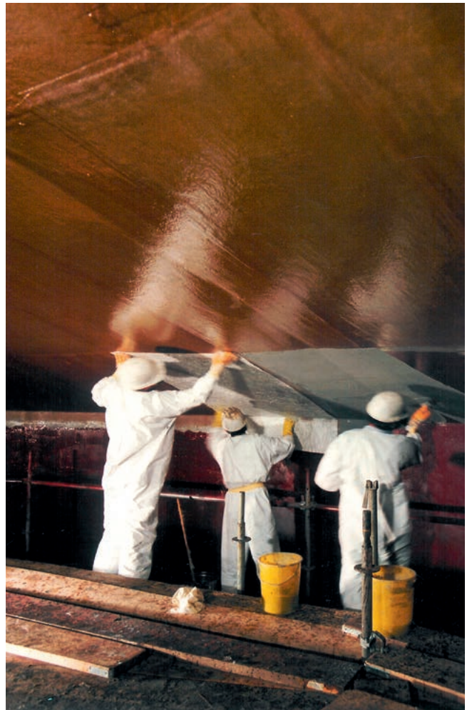
Installing a laminate coating
