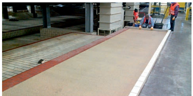
Installing a screed coating
