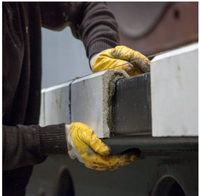
Working with synthetic resin mortar
