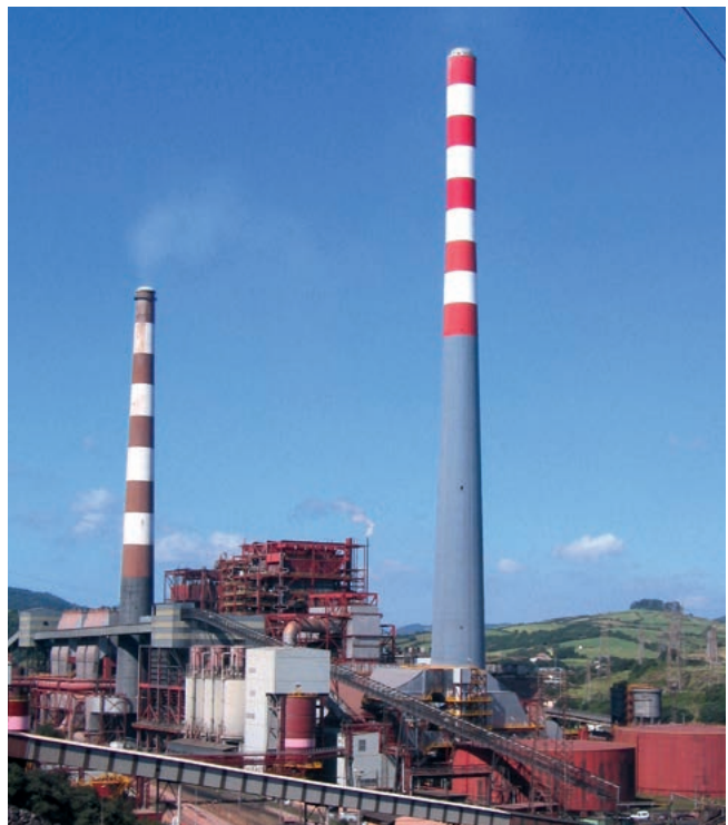
Coated power station chimney
