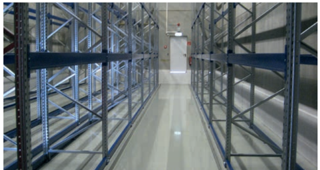
WHG coating in a shelf storage warehouse
