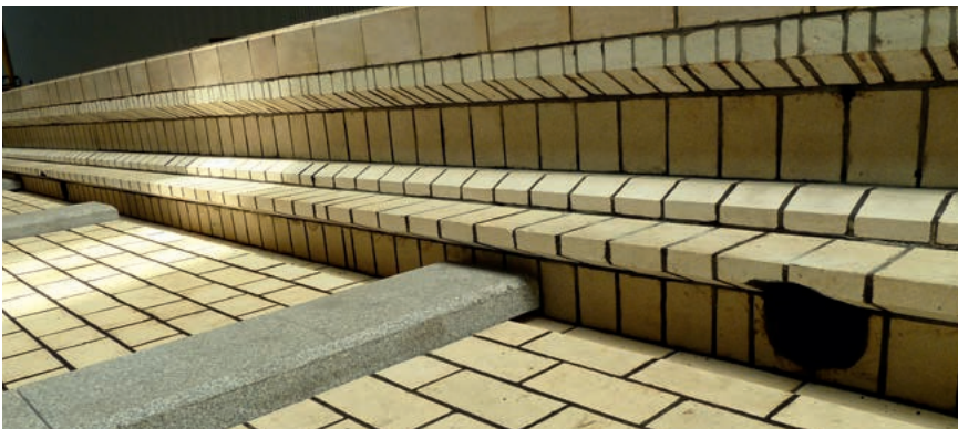
HCl pickling tank lined with ceramic bricks and CHEMOKITT FU 1310
